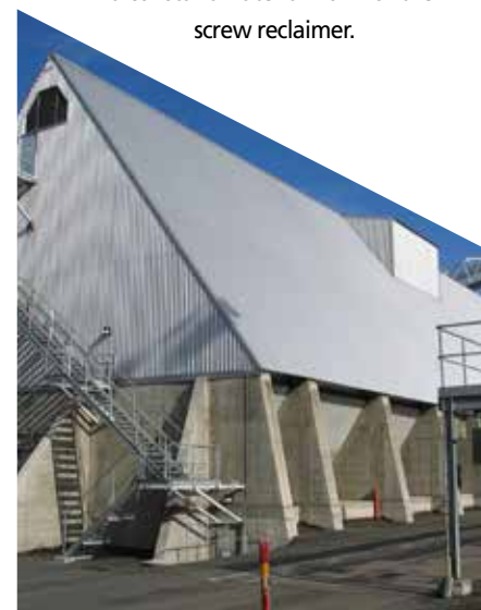
A-frame storages are the most efficient storage systems for maintaining an even fuel quality.
