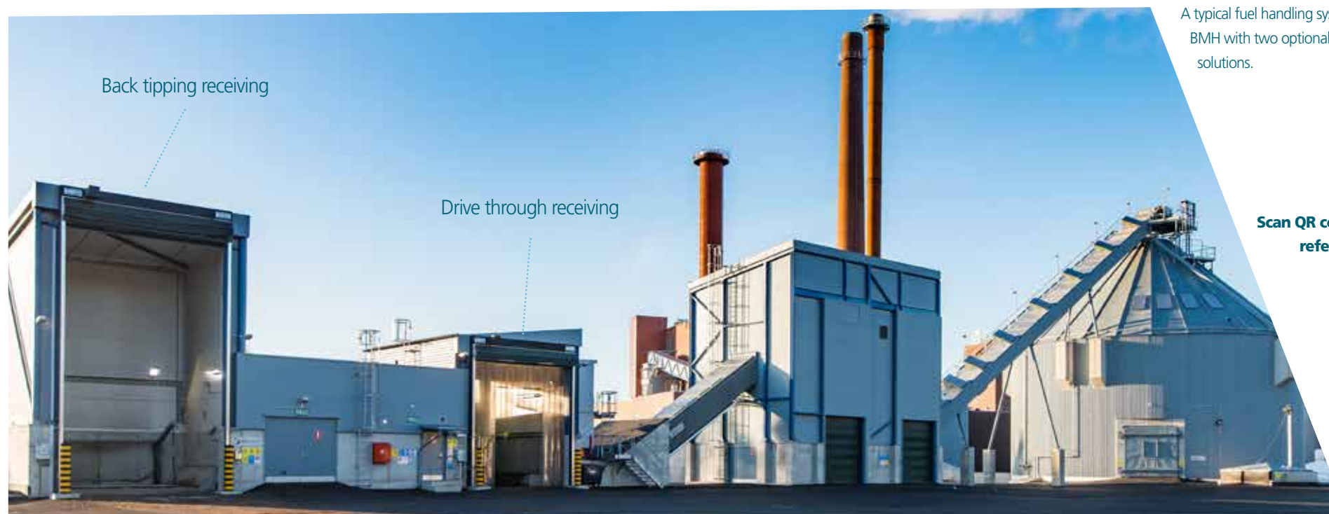
An overdrive reclaiming table is a combination of a fuel storage and a receiving station.
